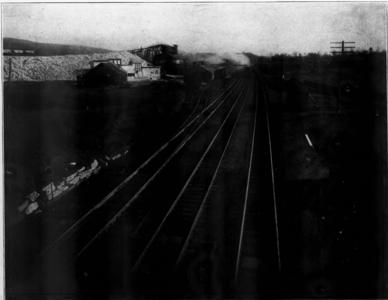
View of Plant Showing Kilns
